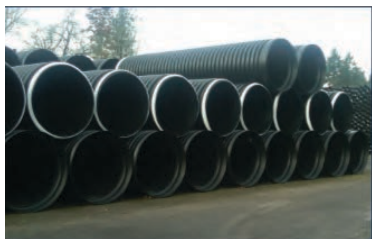
Alternate and offset layers of stacked Bell & Spigot pipe
