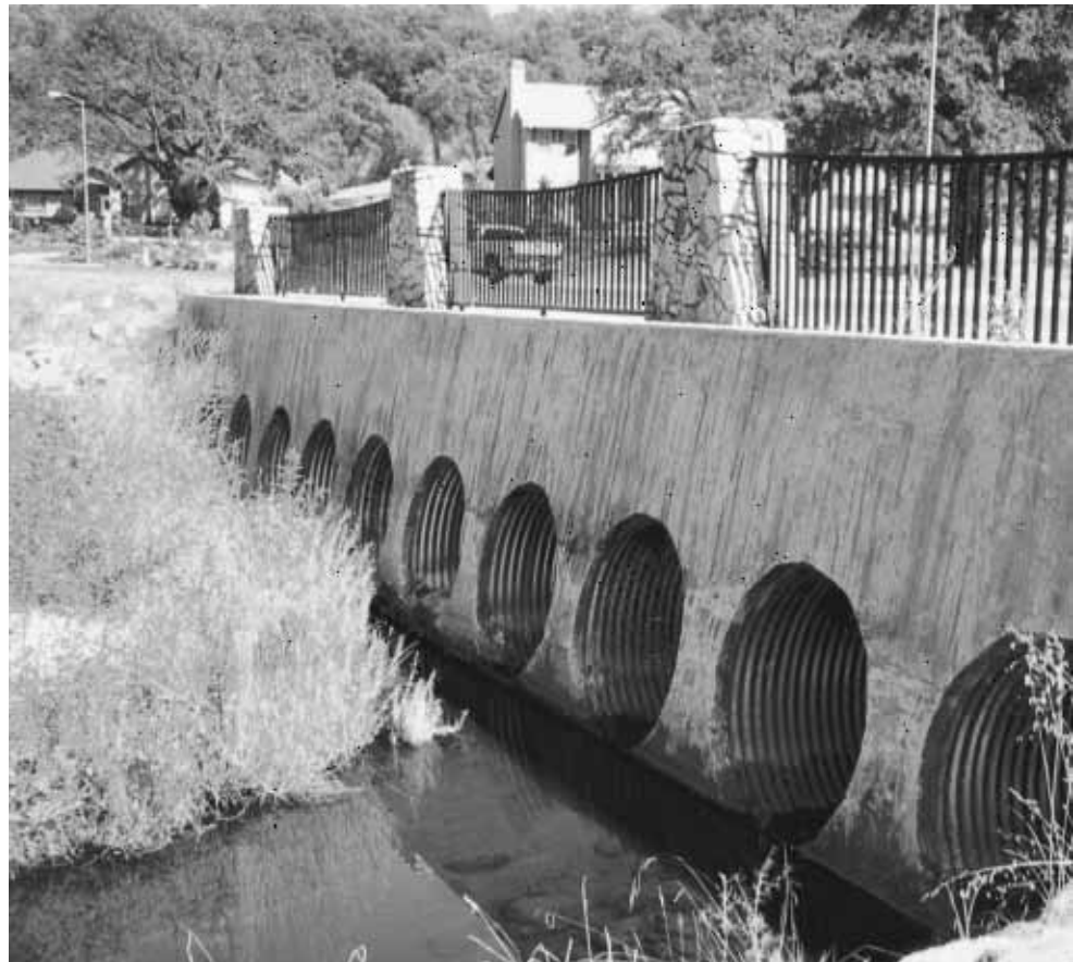
Clove Valley Estates, Rocklin, CA. - Eleven 76 ft. Runs of 60" diameter CSP .064, 3"x1" corrugation
