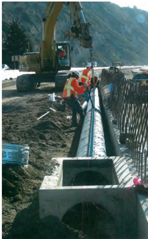
PLACING AND LEVELING SLOTTED DRAIN FROM MANHOLE.
