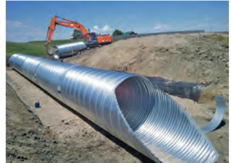
STEP BEVELED END: Our step beveled end pipe is a simple and efficient solution for passages under roadways to control the flow of water. These beveled ends allow for a natural grade to give the installation a more appealing finish.
