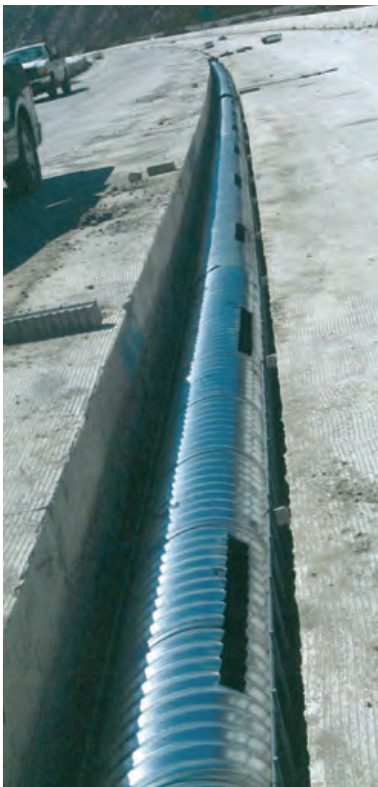
SLOTTED OPENING FOR UNDER ROADWAY BARRIER APPLICATIONS.
