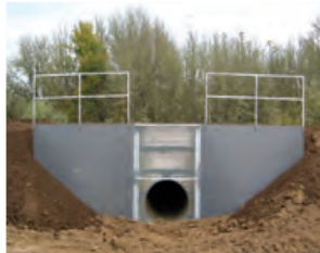
FLASHBOARD RISER WITH GRATING COVER AND WING WALLS
